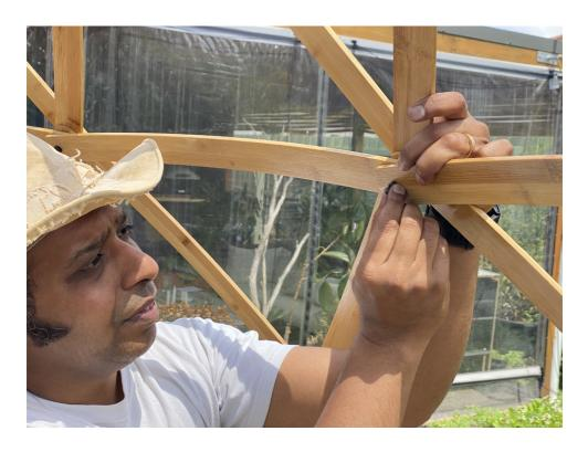
Tighten the bolts using allen key and a spanner. Make sure not to overtighten the bolts as the strength of the structure is not dependent on tight bolts.
