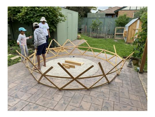
While connecting the last few six dot strips the structure will need to be lifted and stood up.
