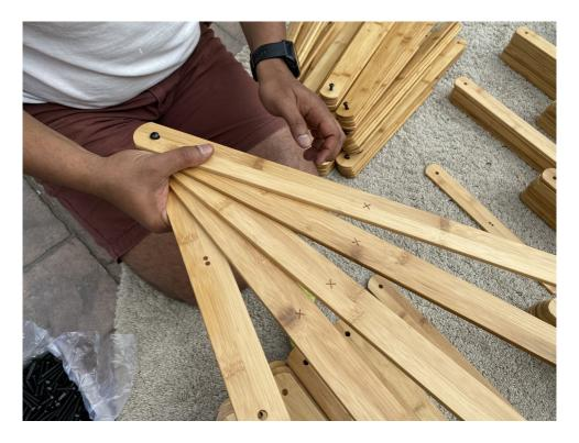
We have found that bundinling some of the strips at the start can simplify and quicken the installation process.
