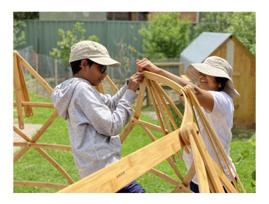
Keep connecting the bundles and tightening the bolts by hand. It helps to have one person on the inside and one on the outside.
